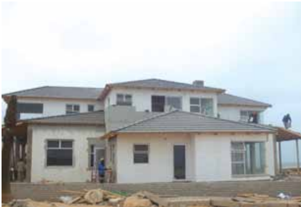
Plumbing to this house was done by RF trainee
